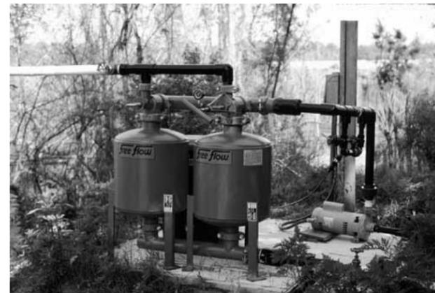
**Sand filter, pump, and fertigation unit**
